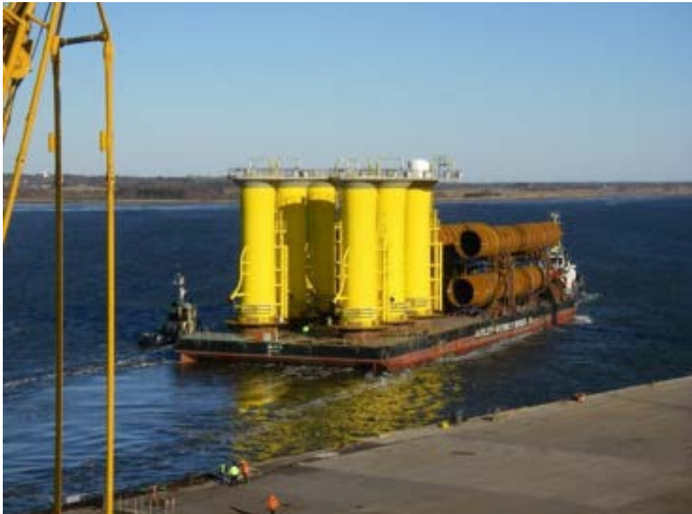
FIGURE 11.3 MONOPILES AND TRANSITION PIECES SAIL AWAY FROM HARBOR (SOURCE: COWI).
