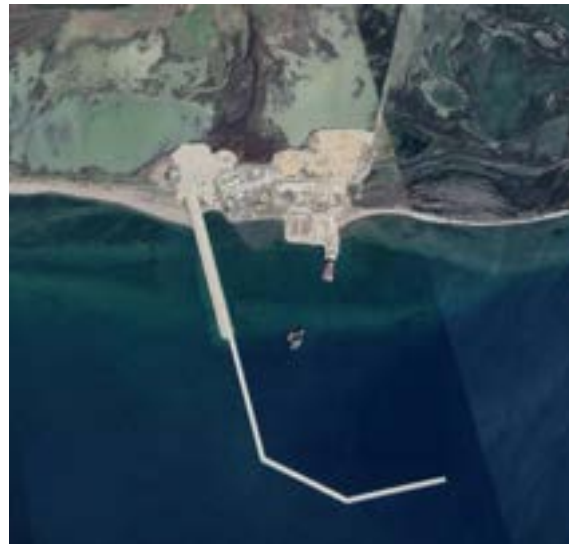
FIGURE 11.9 ÇANDARLI PORT OVERVIEW [80].
