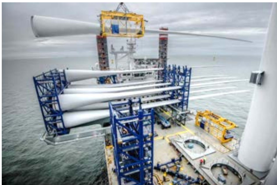
FIGURE 11.2 BLADES EXTENDING OVER THE DECK OF THE WTG INSTALLATION VESSEL [77].
