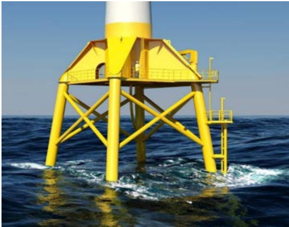
FIGURE 12.8 JACKET STRUCTURE AT WIKINGER (SOURCE: COWI).
