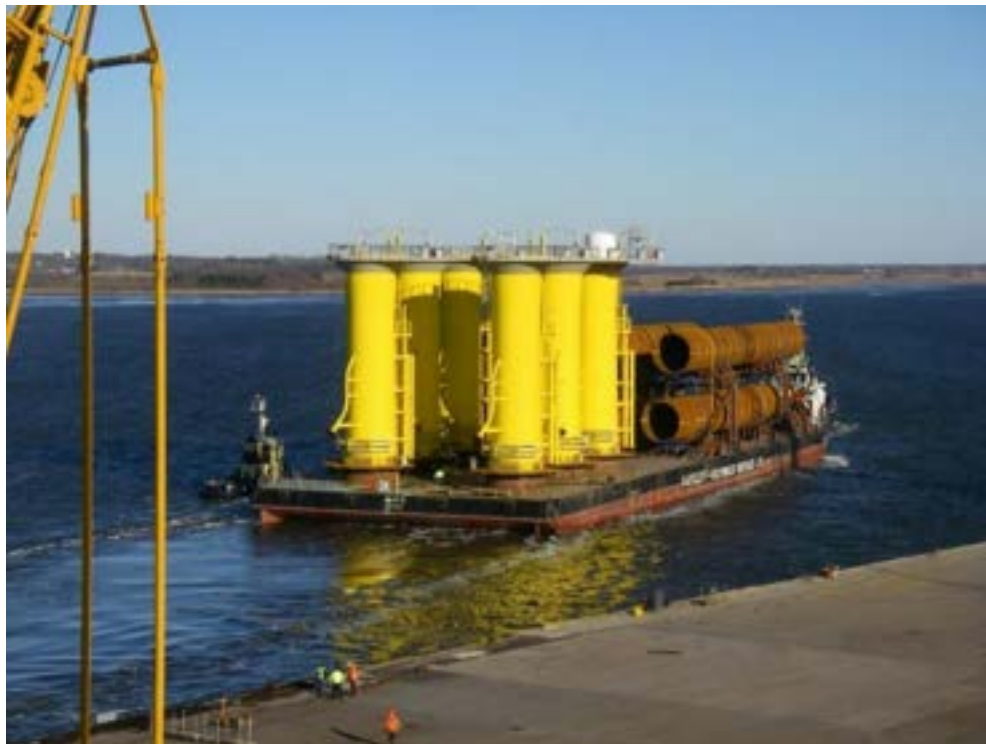
FIGURE 12.7 MONOPILES AND TRANSITION PIECES AT SAIL AWAY FOR LONDON ARRAY (SOURCE: COWI).
