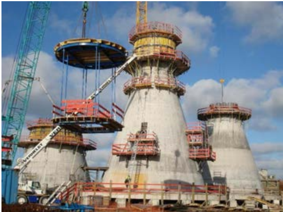
FIGURE 12.6 GRAVITY-BASED FOUNDATIONS FOR THORNTON BANK (SOURCE: COWI).
